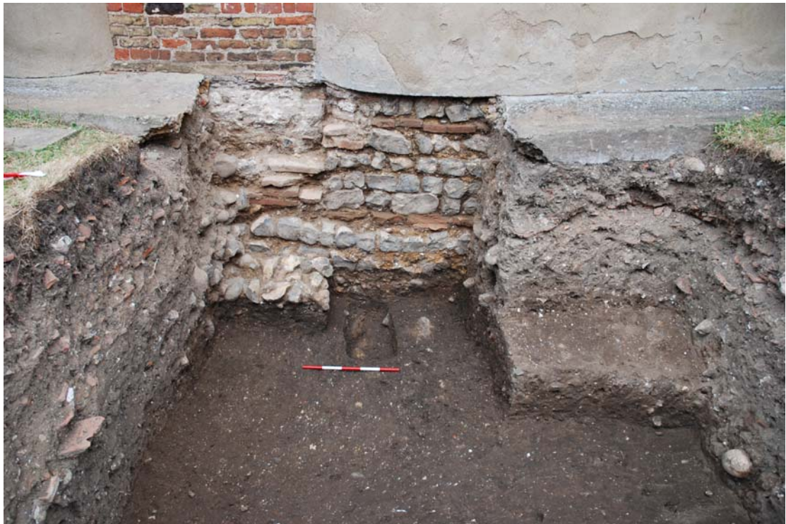
Plate 2 South wall of nave (2049), showing tile string courses and offset foundations
